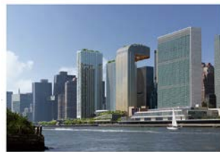
Freedom Plaza river view looking east. Courtesy of Nigata
