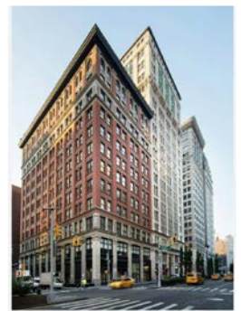
225-233 Park Avenue South
