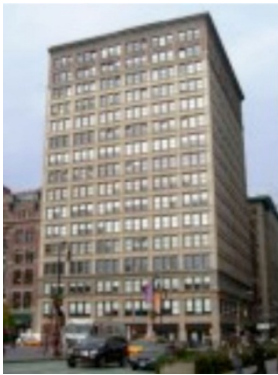
200 Park Avenue South
