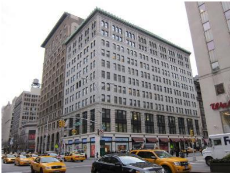
304 Park Avenue South
