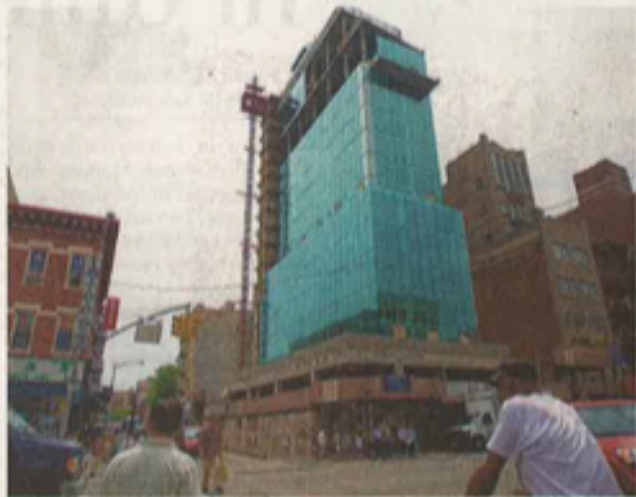
Views of the Wyndham under construction at 91-93 Bowery.
